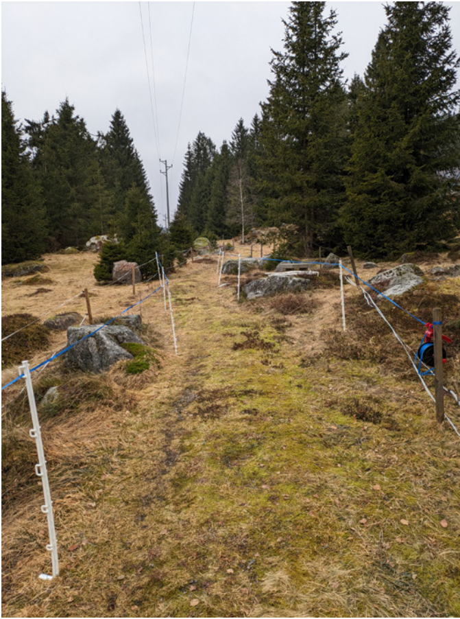
Fig. 3. Setting out the line of a new electric fence (Photo: Rebecca Müller).
